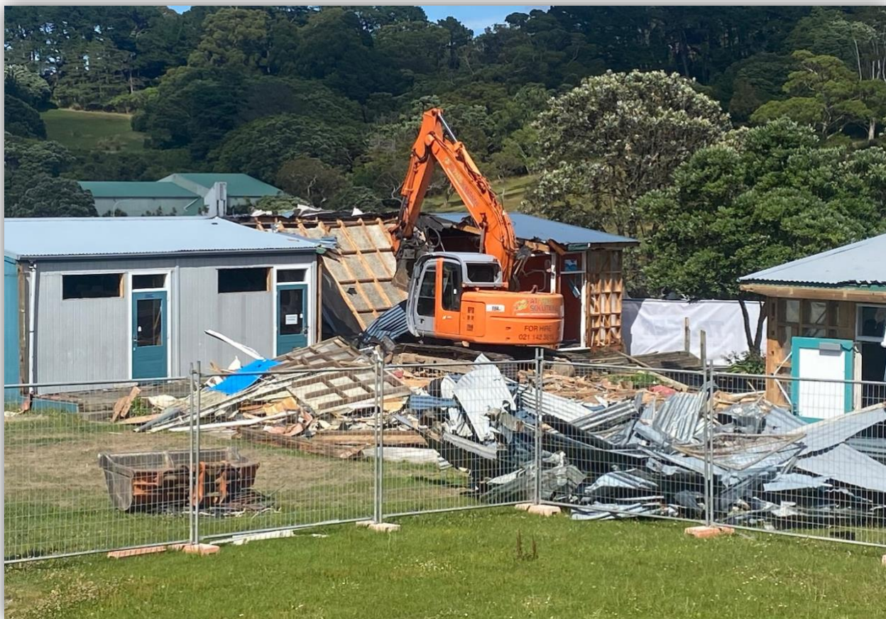
Whātaimai Hub demolition.
